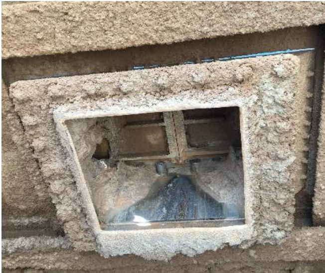
FORMER BULK HANDLING SOLUTION
